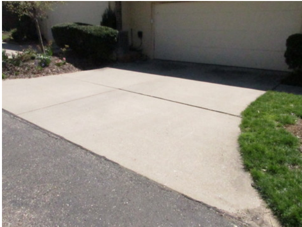
Concrete driveway near Mulberry Lane
