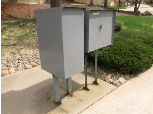
Mailbox station rust
