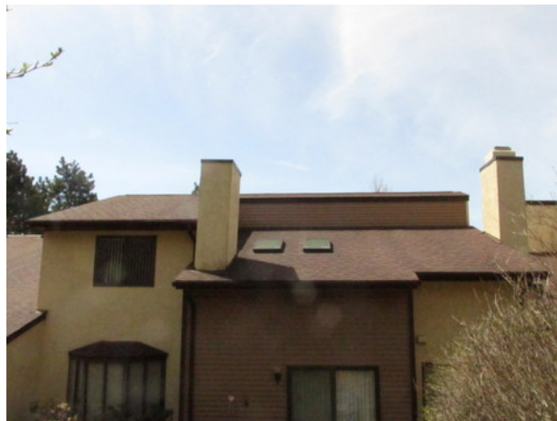
Asphalt shingle roof with skylights
