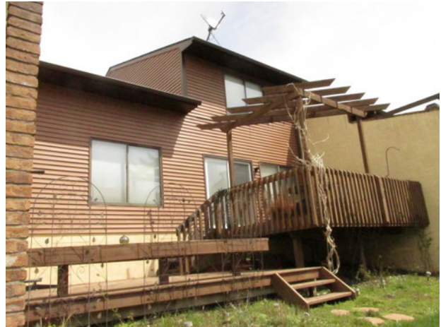
Vinyl siding at rear elevation
