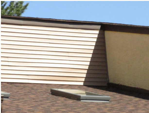
Vinyl siding warp at Unit 94
