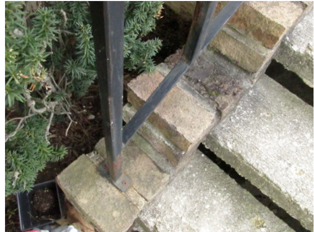
Typical metal railing rust
