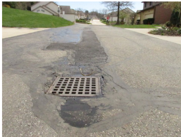
Asphalt pavement street partial replacements and minor catch basin settlement
