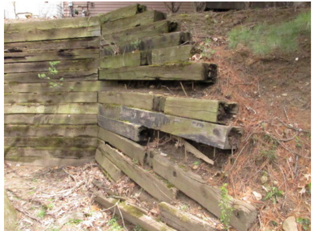
Timber retaining wall damage, lean, board rot, cracks and organic growth
