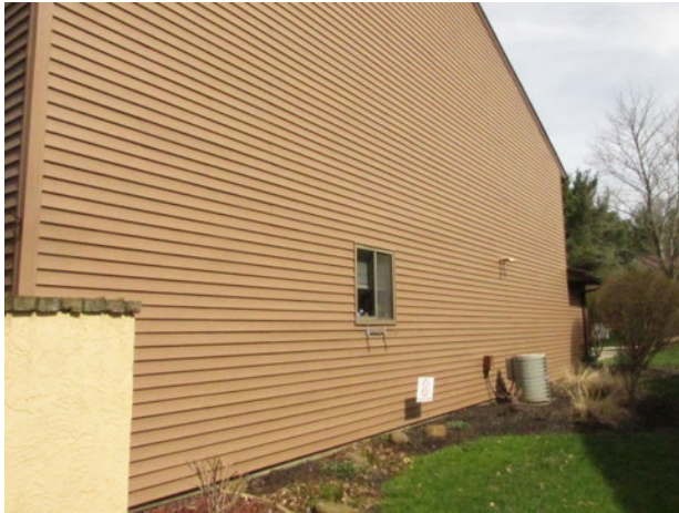
Vinyl siding at side elevation
