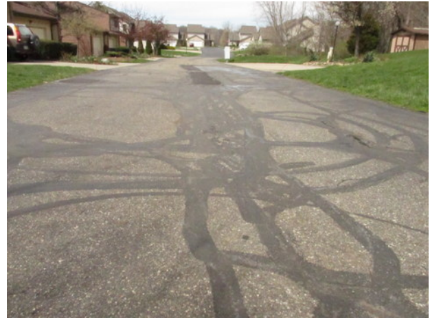
Asphalt pavement street cracks and previous repairs
