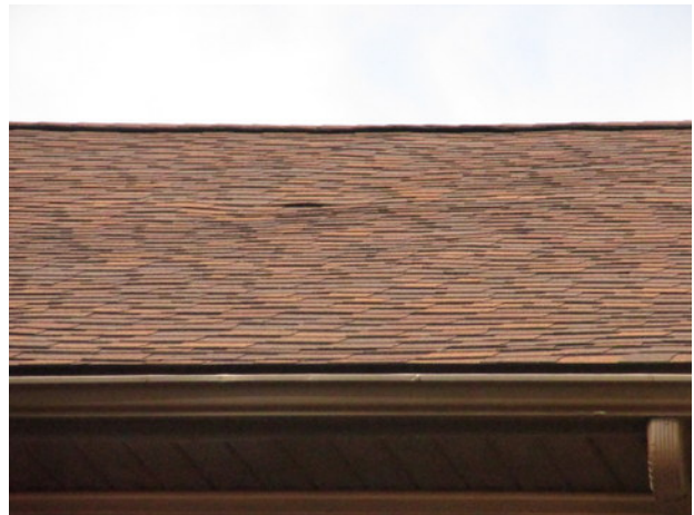
Minor shingle lift near Unit 116
