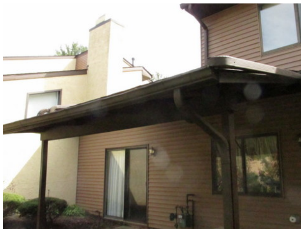
Typical gutter and downspout configuration
