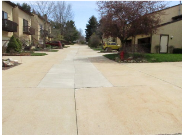
Concrete street partial replacements
