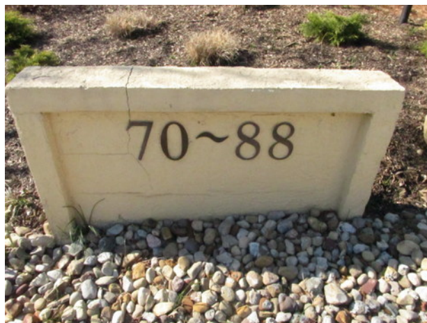
Concrete unit identification signage with cracks
