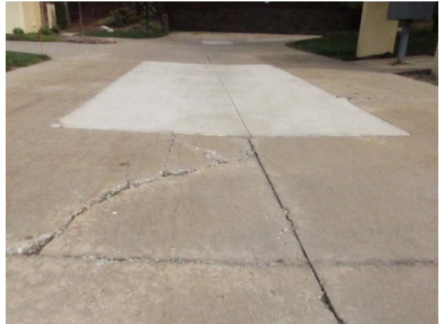
Concrete street cracks, deterioration and partial replacements
