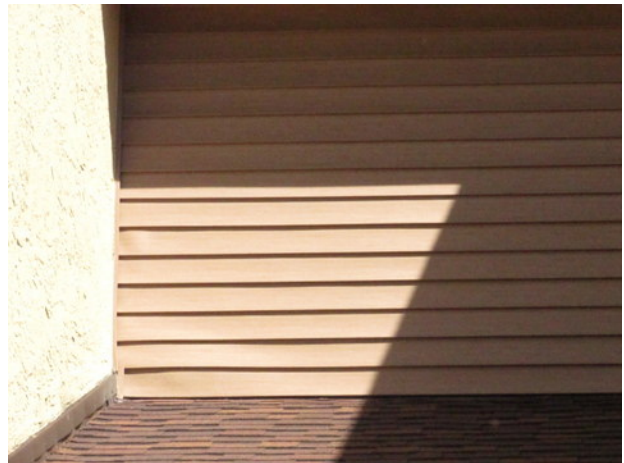
Vinyl siding warp at Unit 70
