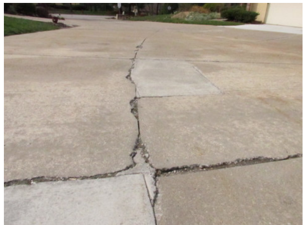
Concrete street settlement, cracks, deterioration and partial replacements
