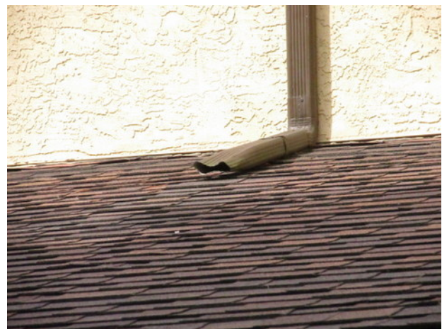
Downspout damage, minor asphalt shingle granular loss and direct downspout discharge onto asphalt shingle roof
