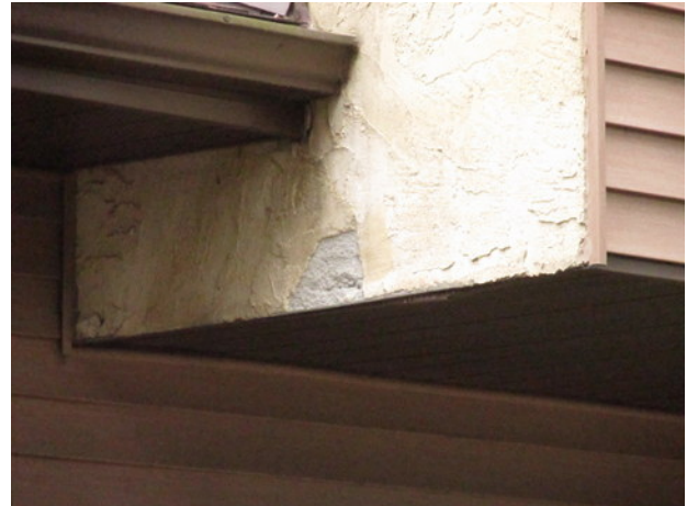
Stucco paint finish deterioration near Unit 76
