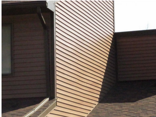
Vinyl siding warp at Unit 131
