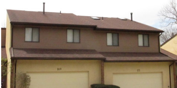
Asphalt shingle roof overview
