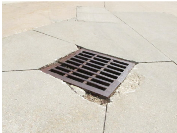
Catch basin with minor settlement
