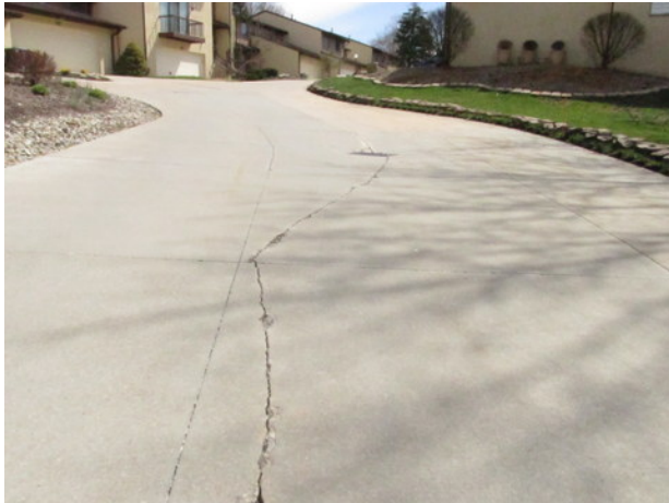
Concrete street cracks
