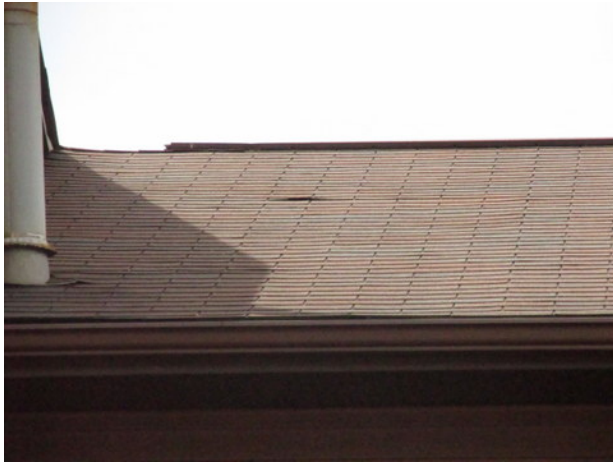
Minor asphalt shingle lift
