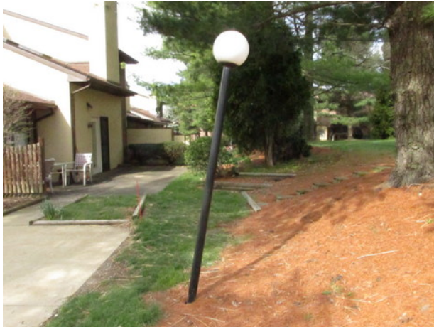
Light pole and fixture with lean
