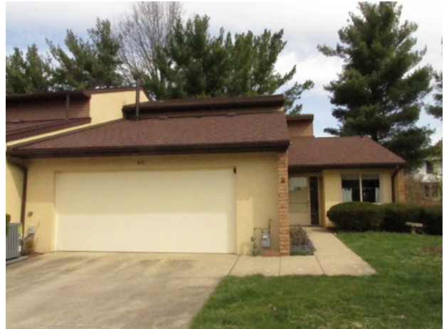
Asphalt shingle roof overview
