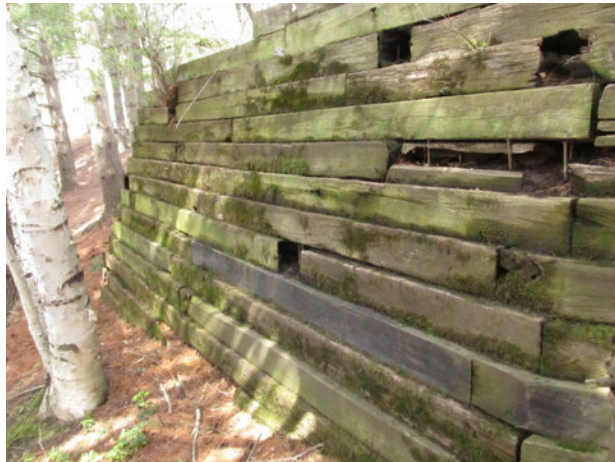
Timber retaining wall lean, rot, cracks and organic growth
