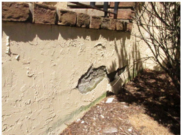
Stucco paint finish deterioration at concrete staircase at Unit 166
