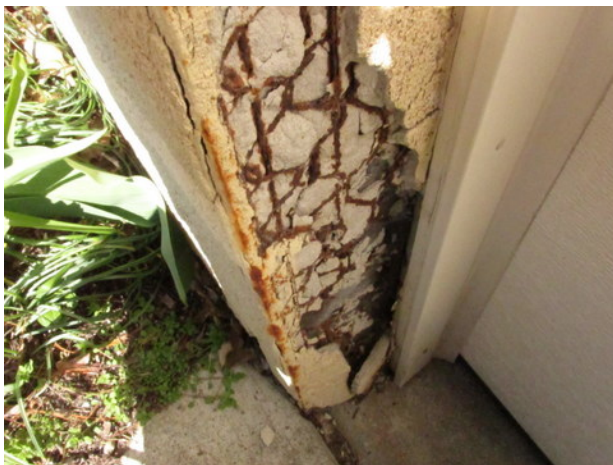
Stucco deterioration near garage door at Unit 70
