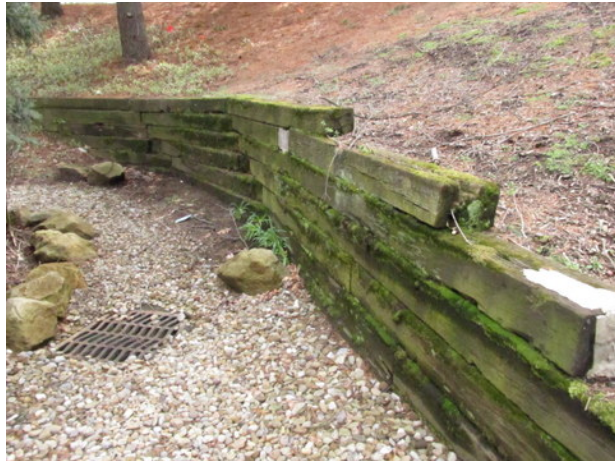
Typical timber retaining wall with lean and organic growth
