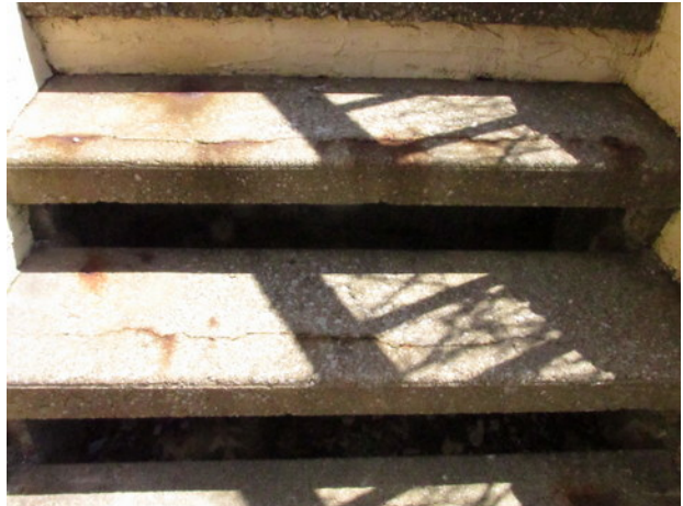
Concrete step cracks at Unit 170
