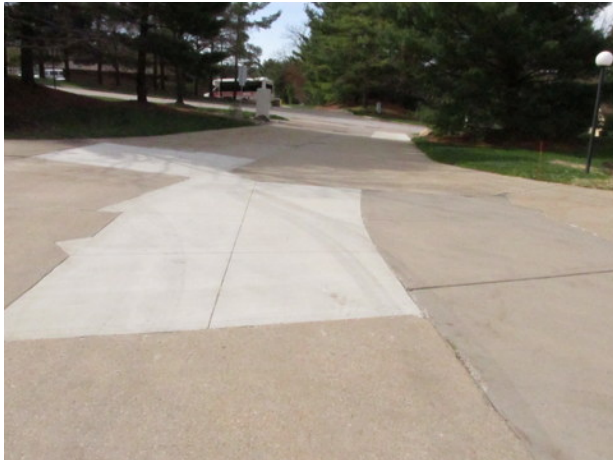
Concrete street partial replacements
