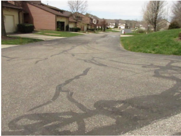
Asphalt pavement street with cracks and previous repairs
