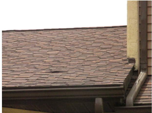
Minor asphalt shingle lift
