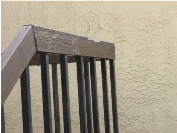
Wood paint finish deterioration
