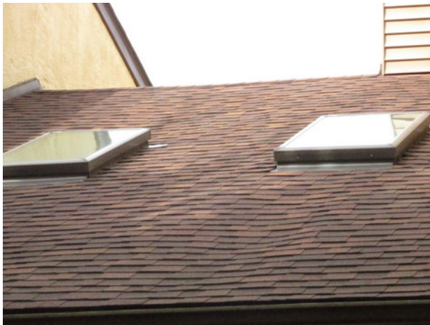
Minor sheathing deflections near skylight at Unit 76
