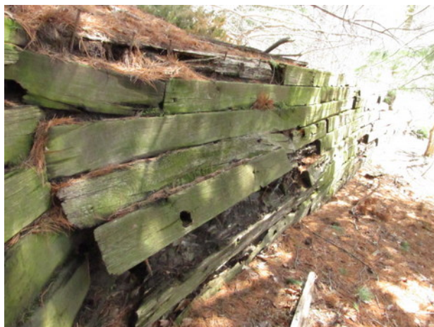
Timber retaining wall lean, rot, organic growth and cracks
