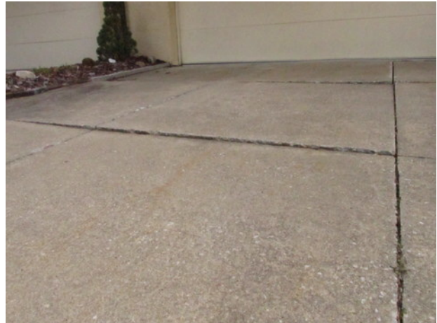
Concrete driveway settlement
