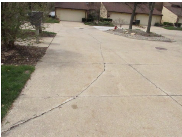
Concrete street cracks
