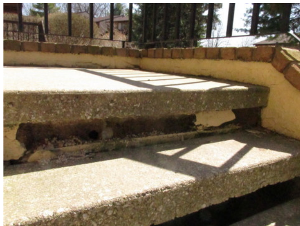
Concrete and stucco paint finish deterioration near landing at Unit 164
