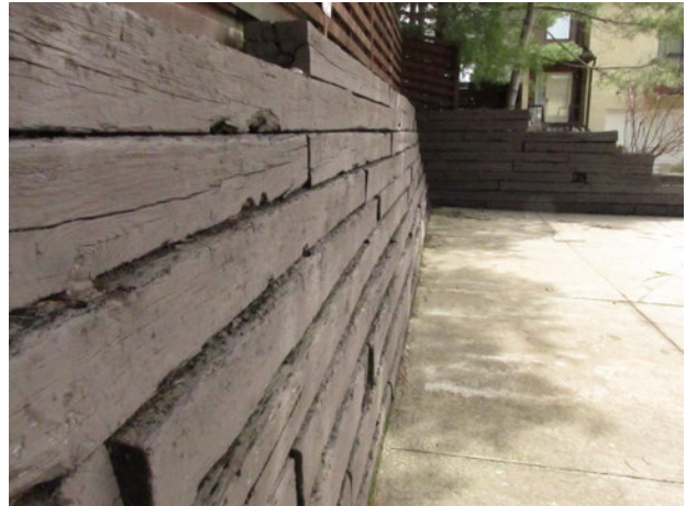
Retaining wall between Buildings 3 and 4 with cracks and displacement
