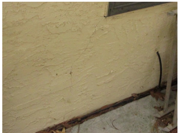
Stucco crack
