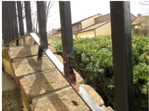
Significant metal railing rust at Unit 114
