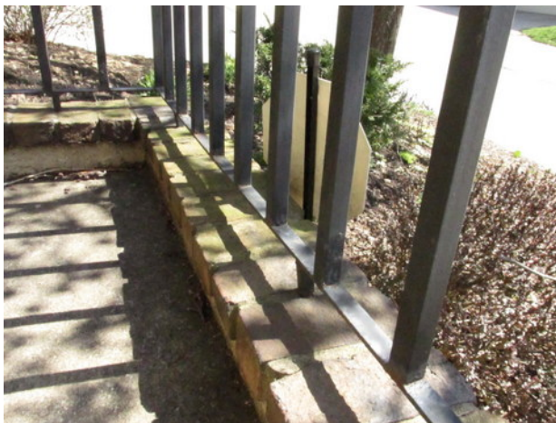
Decorative brick mortar deterioration and organic growth at Unit 130
