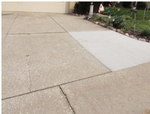
Concrete driveway cracks and partial replacements near Unit 86
