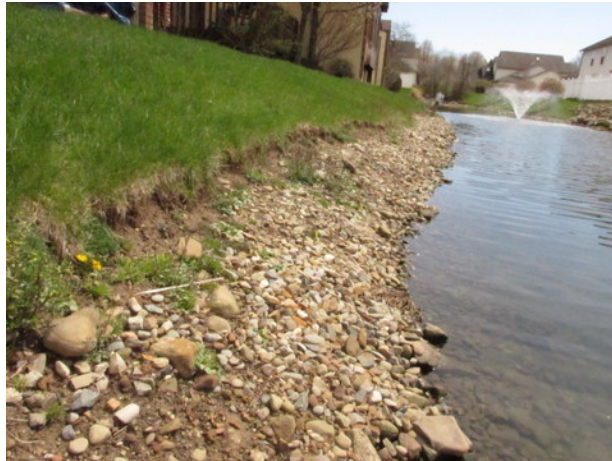
Pond shoreline with minor erosion
