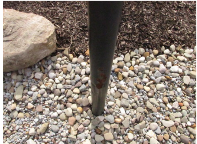
Light pole rust
