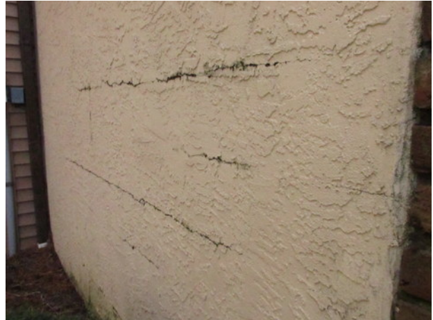
Stucco cracks at Building 10
