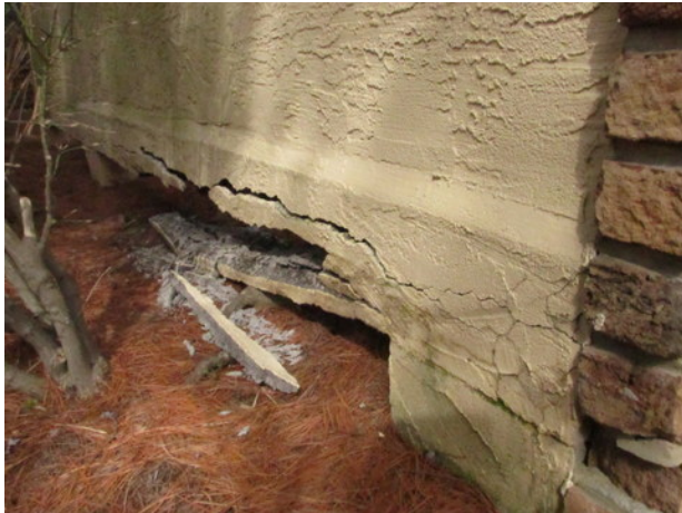
Significant stucco deterioration and cracks at free standing wall near Unit 106
