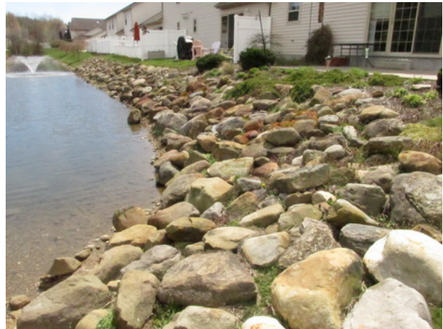
Pond shoreline rip rap
